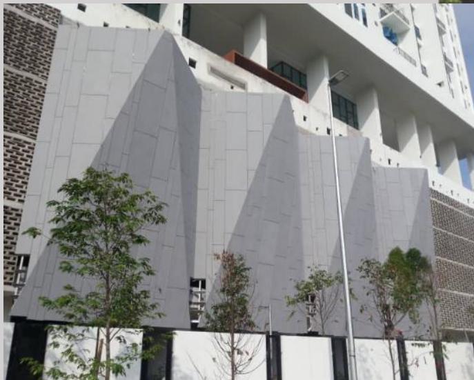
△ Condominium Project in KL ▷ ▪ Design & Install façade framing with combination of mild steel and light gauge proprietary profiles
