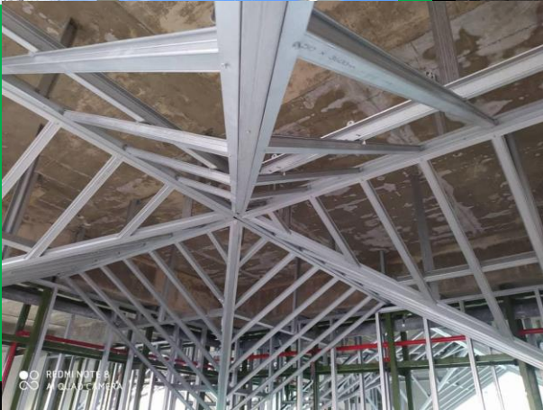
△ Resort in Pulau Tioman ▪ Lightweight building frames ▪ Drywall System ▪ Ceiling System with Plasterboard and Fiber Cement lining
