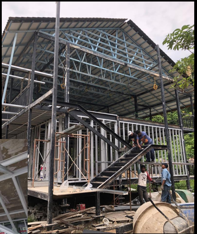
△ Resort in Pulau Tioman ▪ Lightweight building frames ▪ Drywall System ▪ Ceiling System with Plasterboard and Fiber Cement lining
