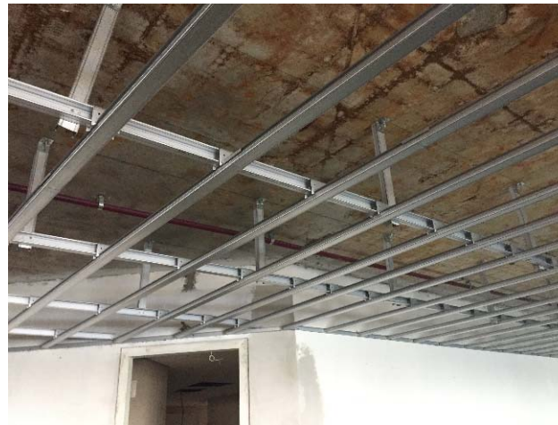
Semi Exposed External Ceiling frame
