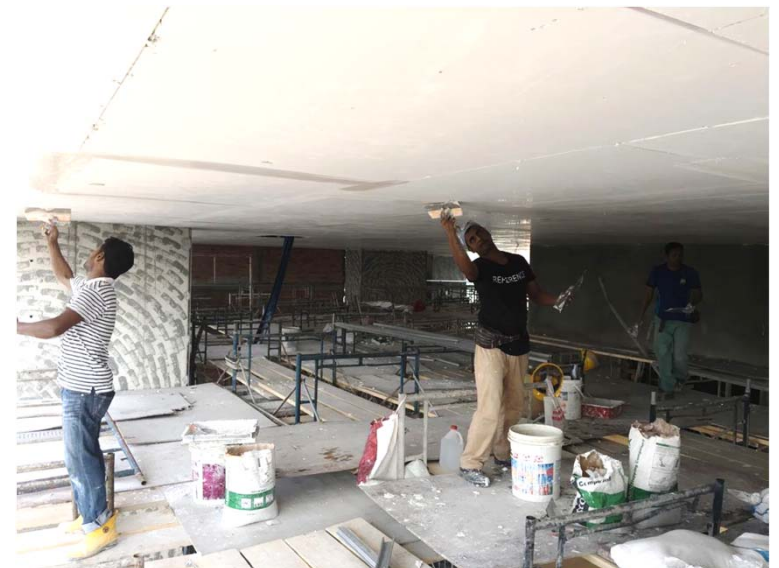
Semi Exposed External Ceiling frame with plasterboard installed
