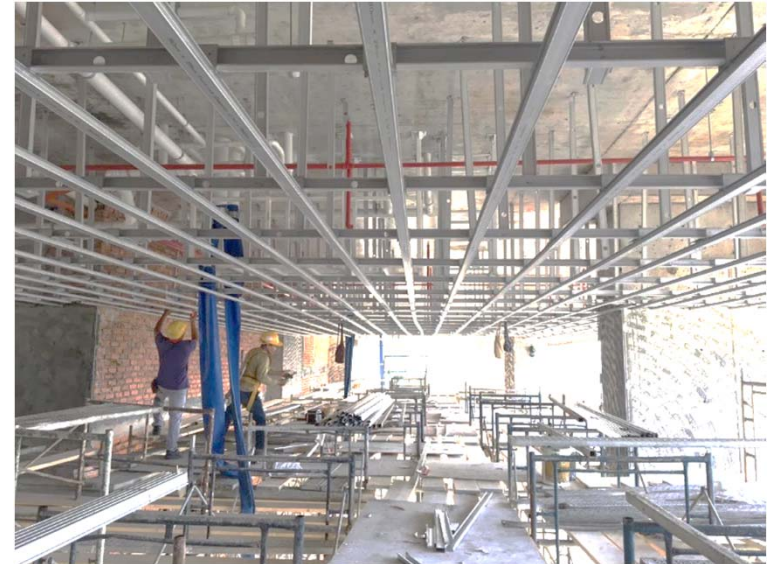
Semi Exposed External Ceiling frame
