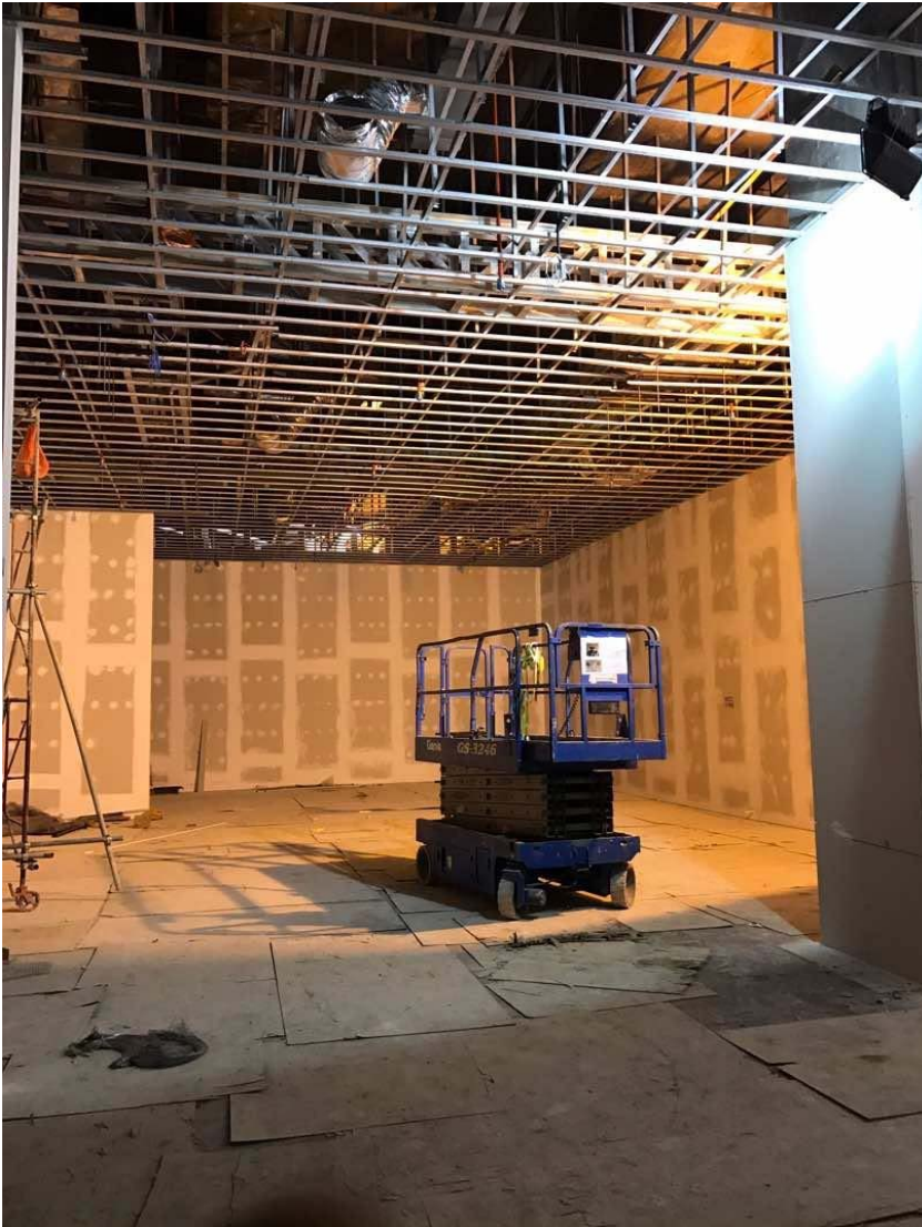
Heavy Duty Ceiling frame with multi layers plasterboard acoustic ceiling system
