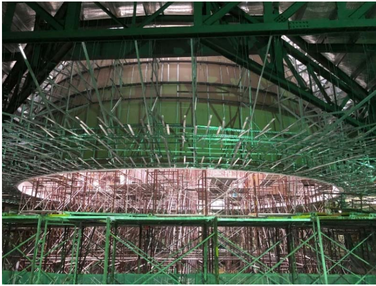
Pre Curved RHS ring beam & Pre Curved furring channel to form Dome ceiling with 2 layer plasterboard
