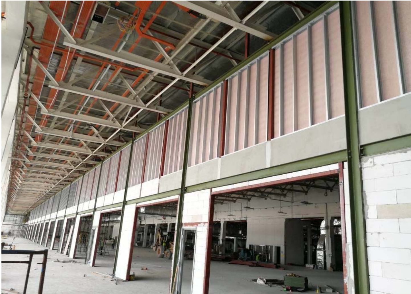
External Drywall frame cladded with 9mm thick Fiber Cement sheet
