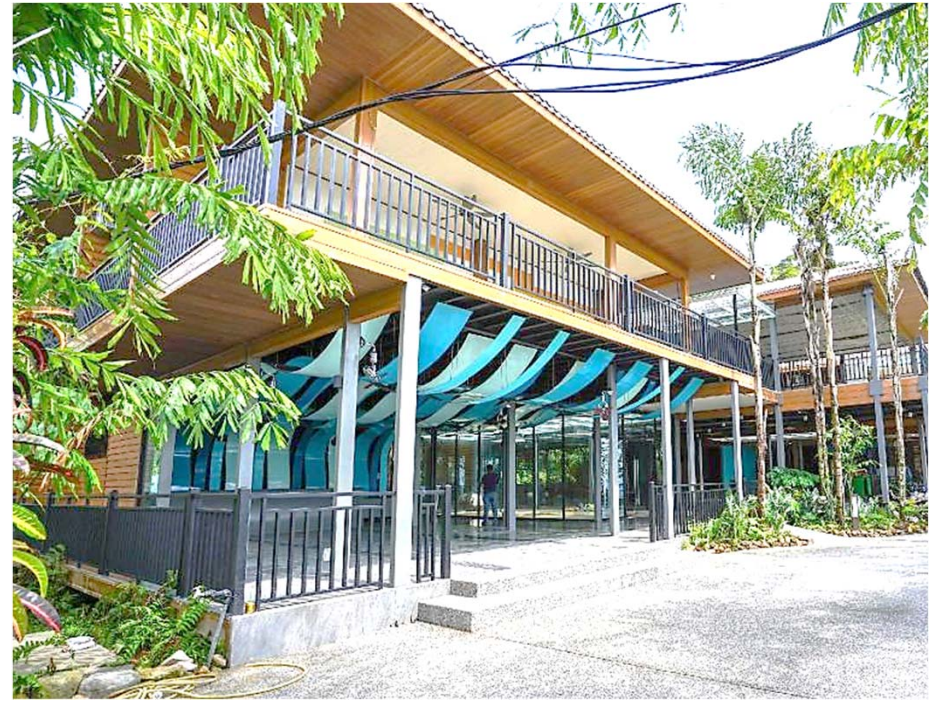
Wave ceiling with Aluminium Panel
