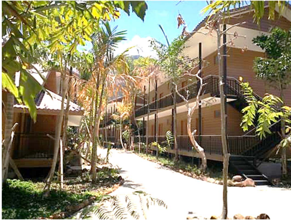
Completed 14 blocks of Chalet with Drywall frame
