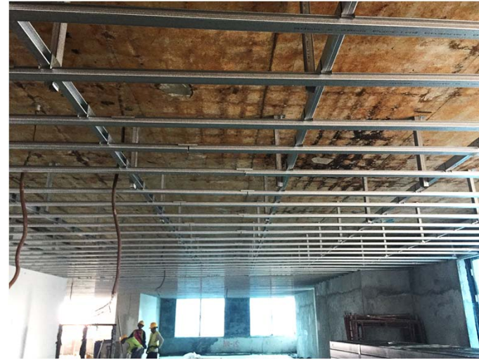
Semi Exposed External Ceiling frame
