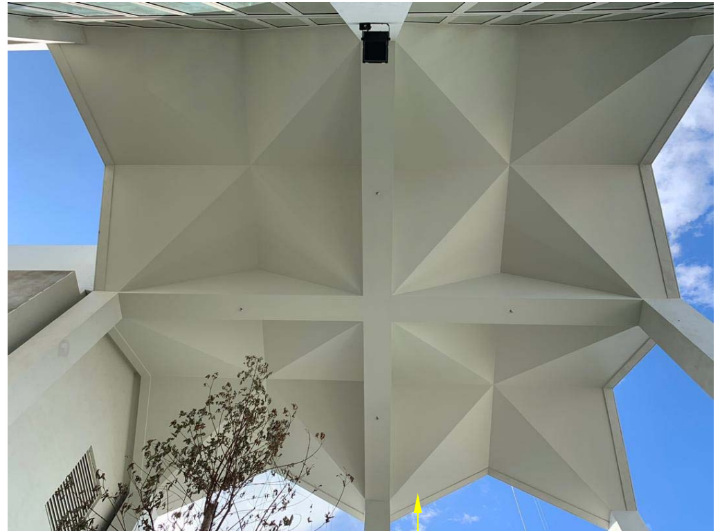
Completed External Ceiling
