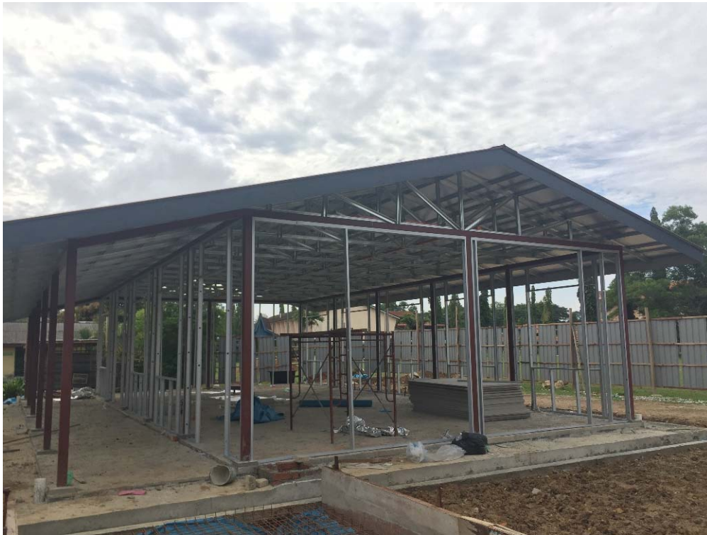
External Drywall frame cladded with 9mm thick Fiber Cement sheet
